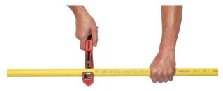
**6.** Cut the pipe to the required length with the recommended multi-layer pipe cutters.
